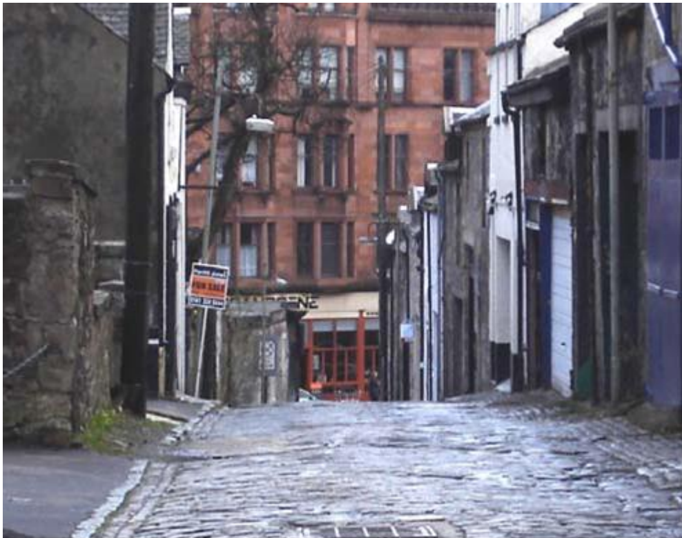
Woodside Terrace Lane – after
