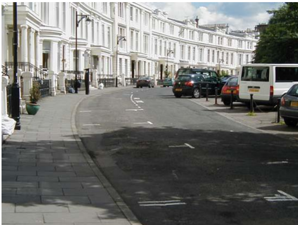
Royal Crescent – after
