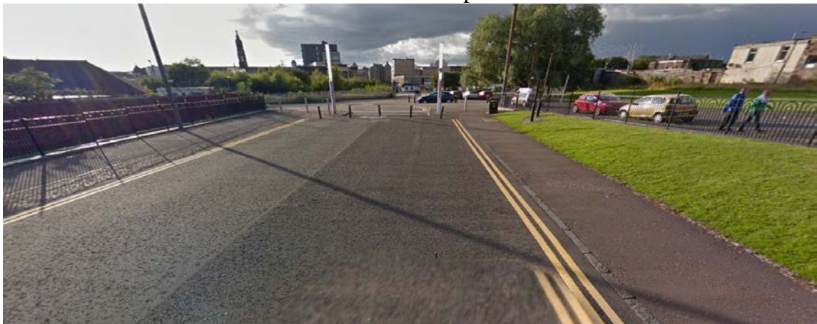
Continue out of the Inspection Area, past barriers onto Greendyke Street
