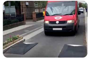
Cycle friendly speed humps – reduce vehicle speed and allow cyclists clear path
