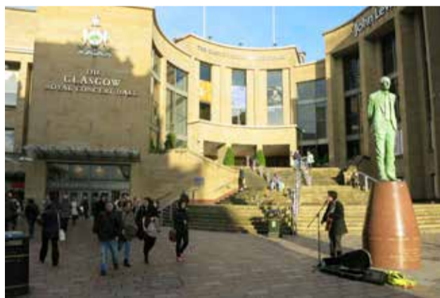
Glasgow Royal Concert Hall has long blank façades and limited entrance points, the public realm doesn't support the cultural experience that the Concert Hall has to offer
