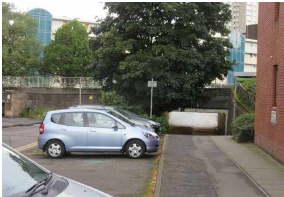
Underpass to Garscube Road at New City Road.
