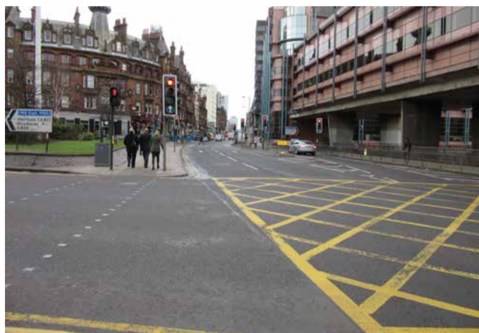
Existing situation. Looking east along Sauchiehall Street at the M8.
