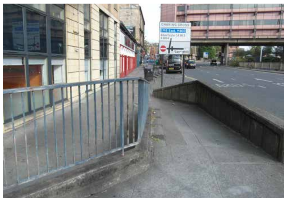
Pedestrian ramp at corner of North Street and Bath Street.
