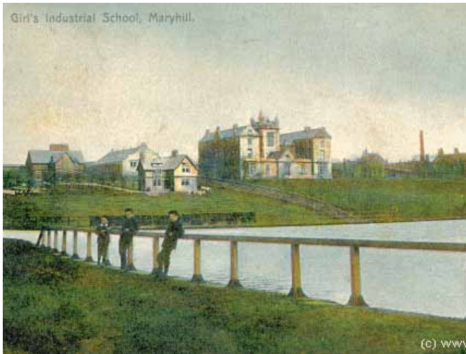
Girls Industrial School overlooking the Forth and Clyde canal
