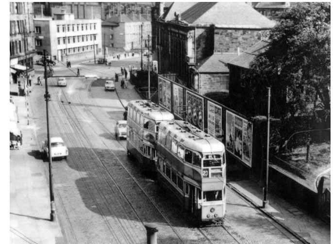
Maryhill Road from canal aqueduct, late 1950s
