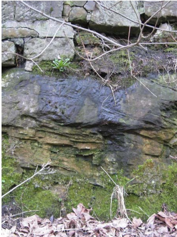
Photo GGS_14 P4: Passage Formation sandstone displaying cross-bedding. The exposure has been partially faced in stone to stabilise the rock face (GGS_14b). Looking E.
