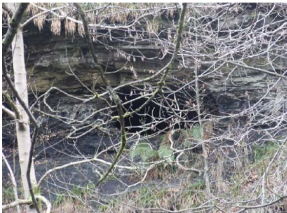
Photo GGS_8 P3: Close-up showing what appears to be void within the sedimentary strata which may be a disused adit in the centre of the image.
