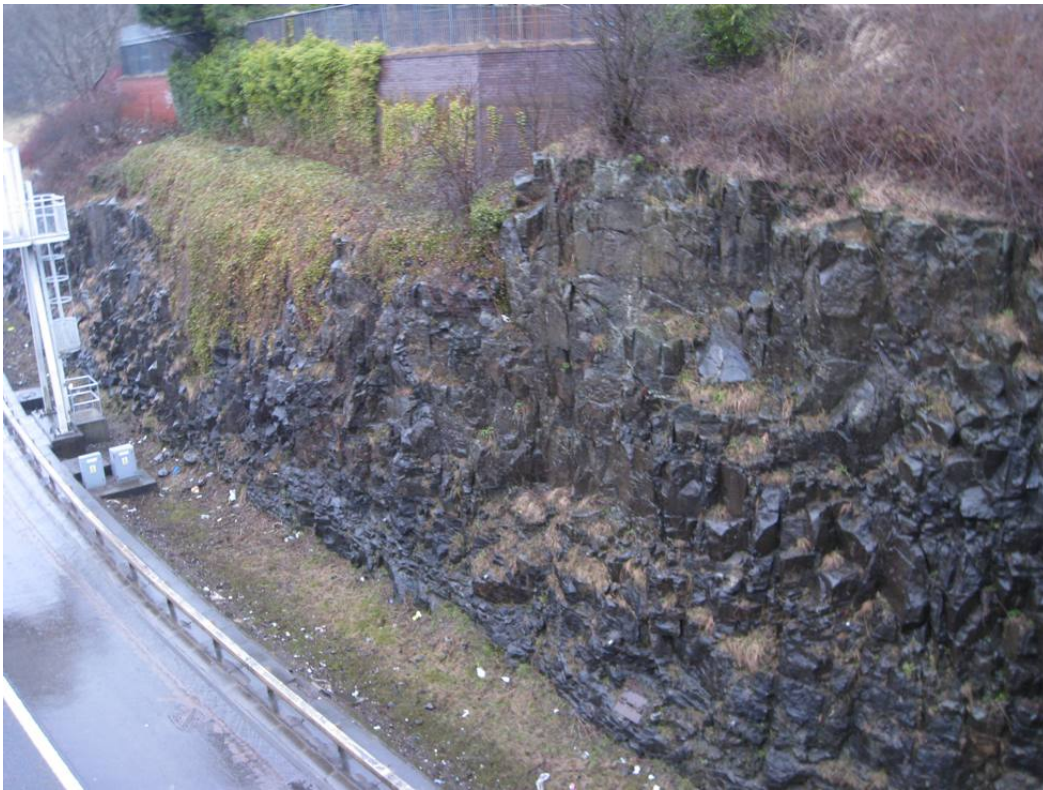
Photo GGS_15_P1: View of M8 road cutting from Gartcraig Road Bridge. Looking NW. Microgabbro sill overlies sedimentary strata of the Scottish Middle Coal Measures Formation. (Note that the exposures can be seen in Street View images on Google Earth)
