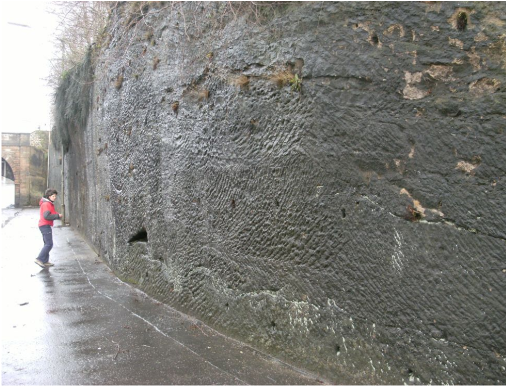
Photo GGS_11 P1: View of Possil Road cutting (GGGS_11a) looking NE, aqueduct located in far left. Massive medium to coarse-grained channelized sandstone unit. Base of channel scours can be seen c. 0.5m and c. 2.5m from the base of the exposure. Tool marks are well preserved on the rock face.
