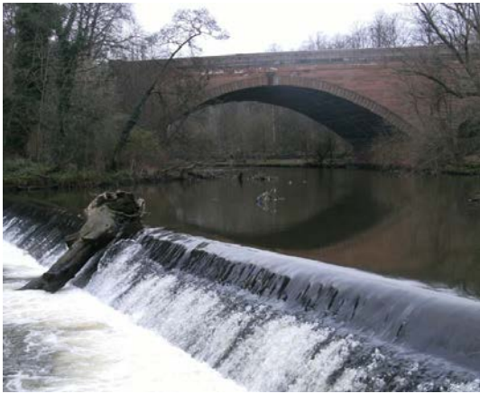
Photo GGS_4 P3: The weir and sluice located immediately downstream of the Queen Margaret Bridge was formerly used to control water entering the mill lade, which carried water to the North Woodside Flint Mill. The bridge, built 1926-1929 is made from concrete but faced with red Corncockle sandstone and solid red Peterhead granite parapets (according to the GCC leaflet on the Botanic Gardens). Looking NW.
