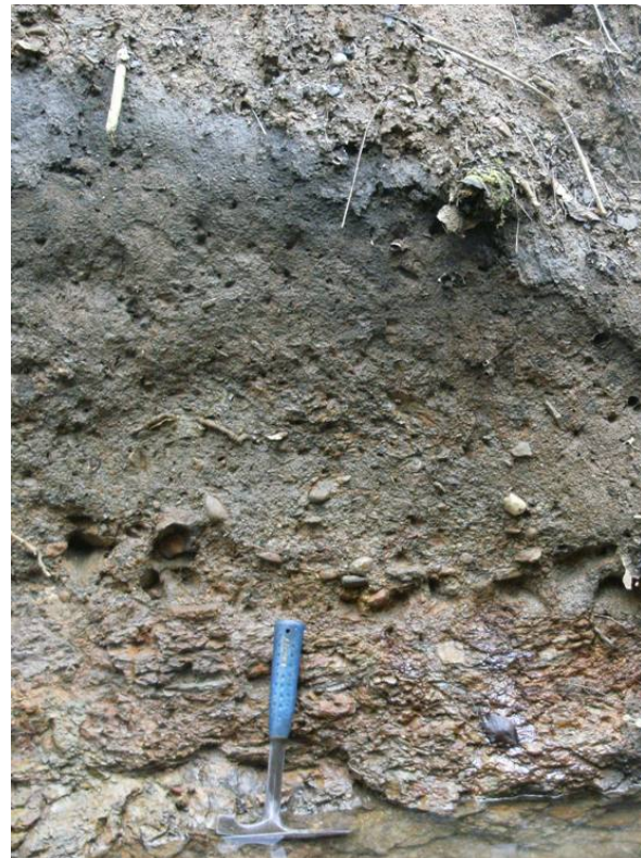
Photo GGS_16_P6: Diamicton (glacial till) overlying siltstone of the Scottish Middle Coal Measures Formation in the Ravel Burn. Contact just above the handle of the hammer. The diamicton is in turn overlain by made ground deposits, visible at the top of the photograph (GGS_16c)
