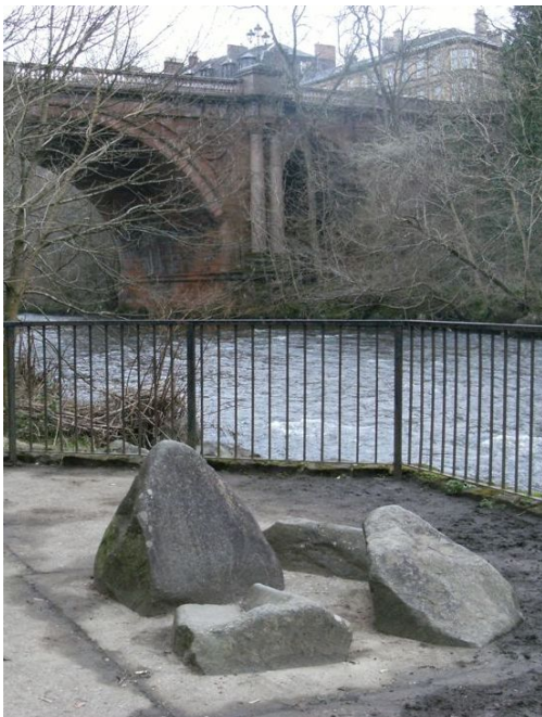
Photo GGS_5 P6: The Kirklee Bridge, built 1899-1900, is constructed of red sandstone with polished pink granite columns and balustrades. In the foreground a number of boulders cemented into the ground form an interesting feature, no explanation for their existence was found. Looking E.
