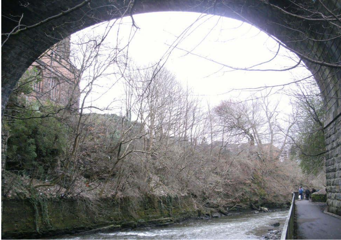
Photo GGS_4 P1: The eastern bank of the River Kelvin, immediately downstream of Belmont Bridge has been stabilised with a concrete facing which prevents erosion occurring on the outside of the river meander, but obscures any potential bedrock exposures. However, further downstream (opposite the people in the photo above) rock outcrops are visible in the bank side, displaying a sequence through the Limestone Coal Formation. Looking SE.
