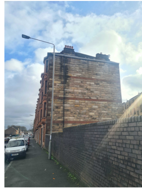
West Facing Façade. Blonde Bullnose Ashlar sandstone.
