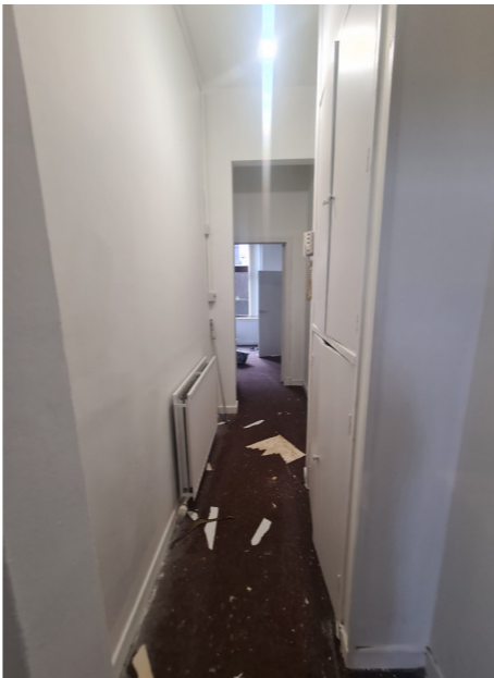
Hallway of flat in building.
