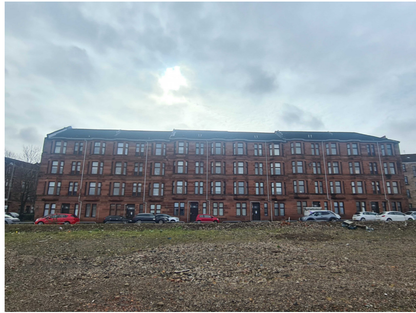
North facing front façade of building. Ashlar red sandstone external walls.
