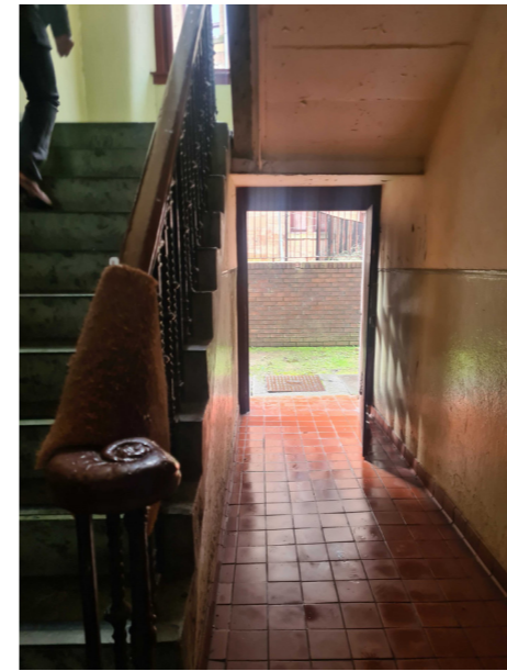
Ground floor communal corridor. concrete flooring with Terracotta tile floor covering. Rear external gate opening up to outdoor garden space.
