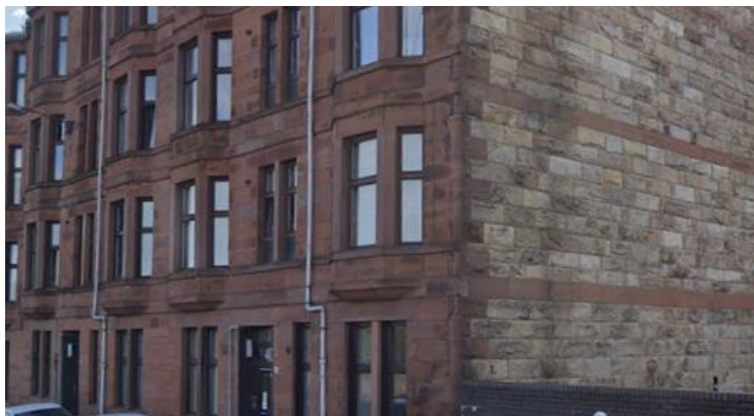
Figure 1. Photograph showing the existing stonework of 40 Old Shettleston Rd
