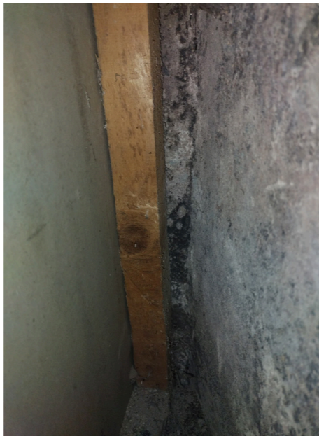
Opening up rear wall showing existing service void behind plasterboard finish.
