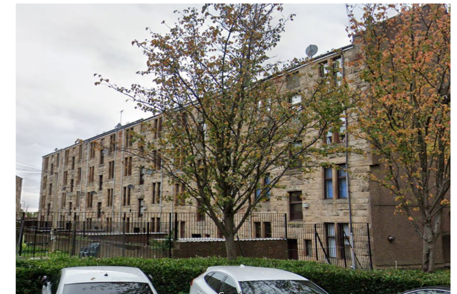
Figure 4 - Rear of existing building with existing outdoor spaces
