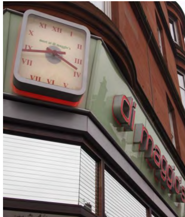
Level 4 High quality traditional and restored frontages that demonstrate a quality and respect for architecture and context
