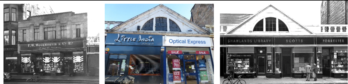
61 Kilmarnock Rd. 1939 (Glasgow City Archive-ref. C6318); 71-73 Kilmarnock Rd. 2015 & 1939 (GCA- C6326)
