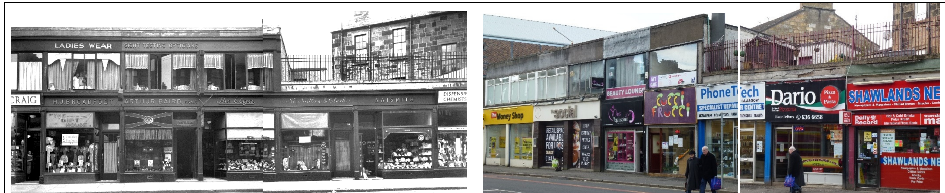
16-34 Kilmarnock Rd. 1939 (Glasgow City Archive-Ref. C6337&8) & 2015 showing dominance of patchwork signage
