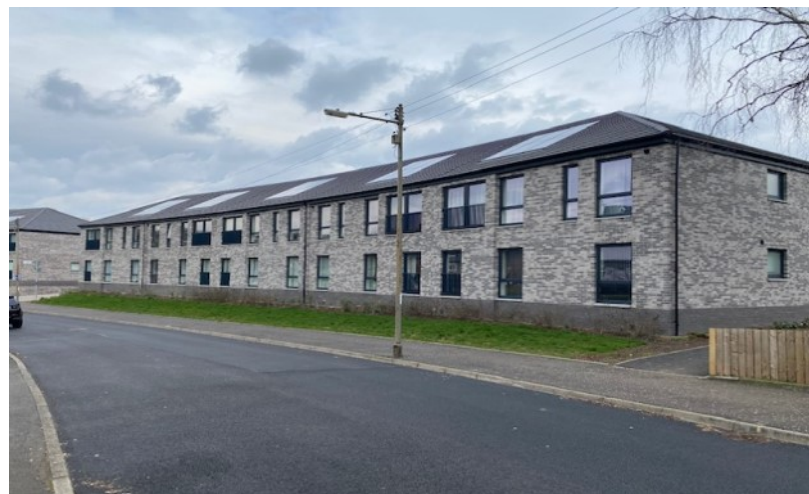
Damshot Road new homes: Old Pollok
