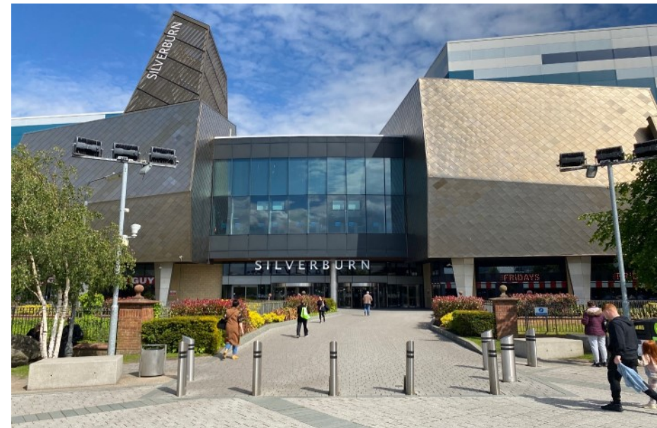
Silverburn Shopping Centre West Entrance
