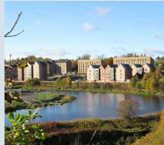
The Canal Partnership with Scottish Canals,
