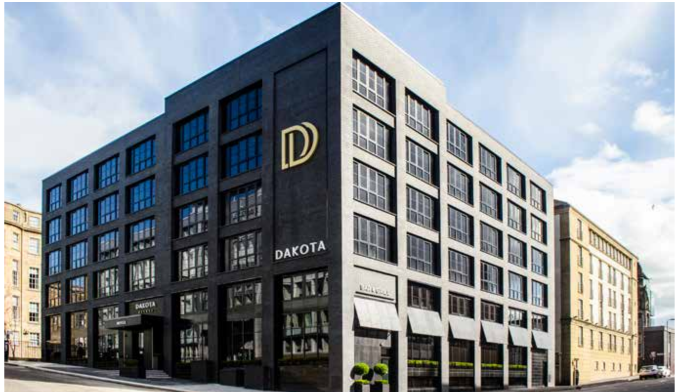
Dakota Hotel (Glasgow Institute of Architects (GIA) Design Awards Winner: Design Award for Commercial.
