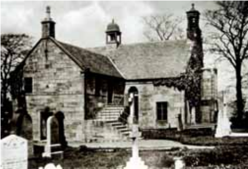
Carmunnock Church (facing north)
