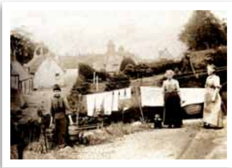
Washerwomen at Pathhead Cottages
