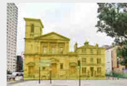
Assess built heritage with historic value
