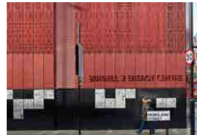
Bunhill Energy Centre - Cullinhanstudio.com
