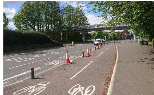
Two-way cycle track (near-completion) – Garscube Road
