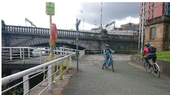
Pinch point and low section under bridge - Shared-use path, unsegregated (Clyde Walkway)
