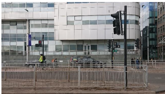
Three-stage 'Toucan' crossing – Broomielaw / Tradeston Bridge
