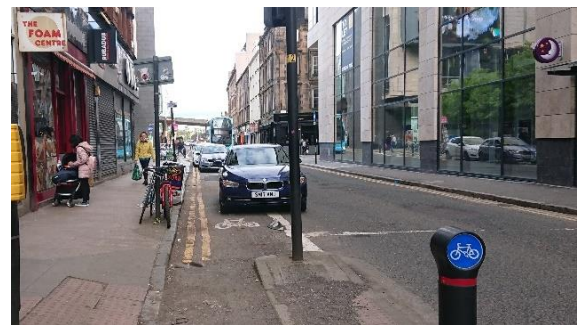
Narrow, poorly maintained and obstructed two-way cycling on one-way street – Howard Street
