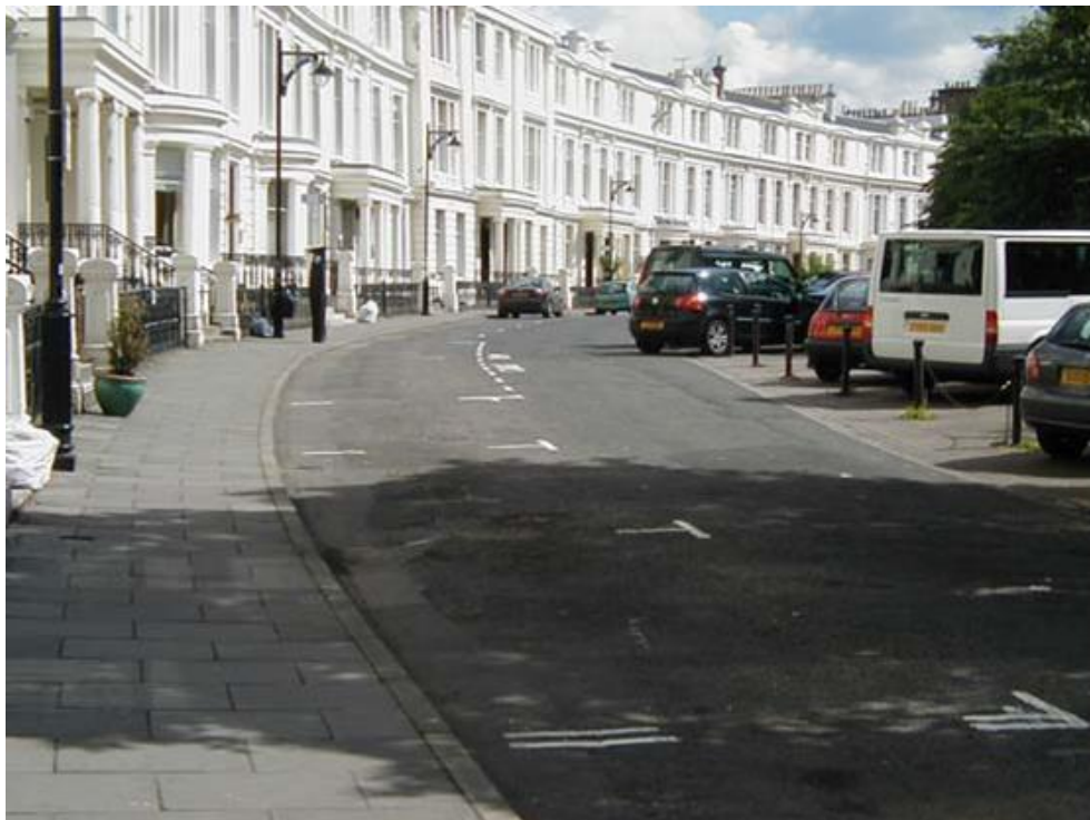
Royal Crescent – after
