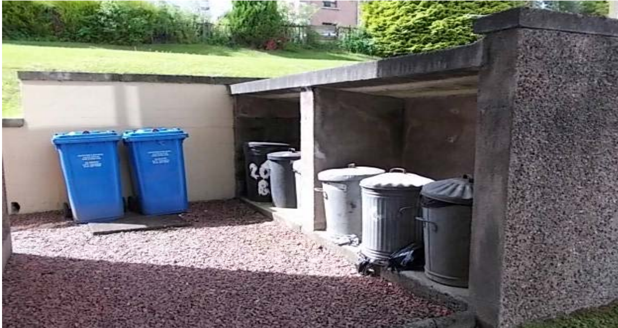
Blue bins within a backcourt
