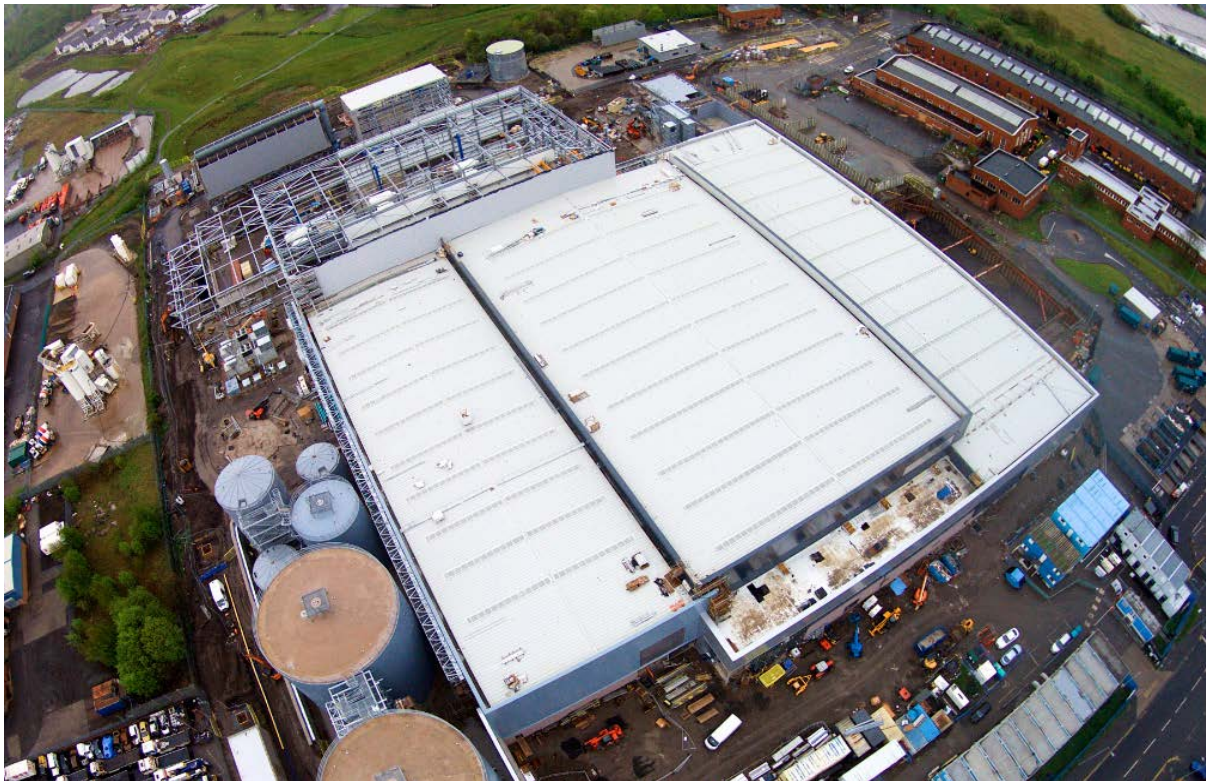
GRREC under construction
