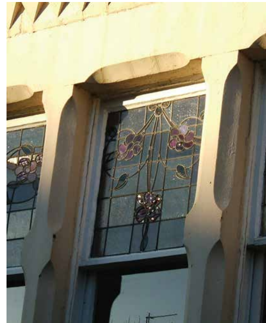
Top left: 'Slimline' double glazing in historic frame and retention of original ironmongery
