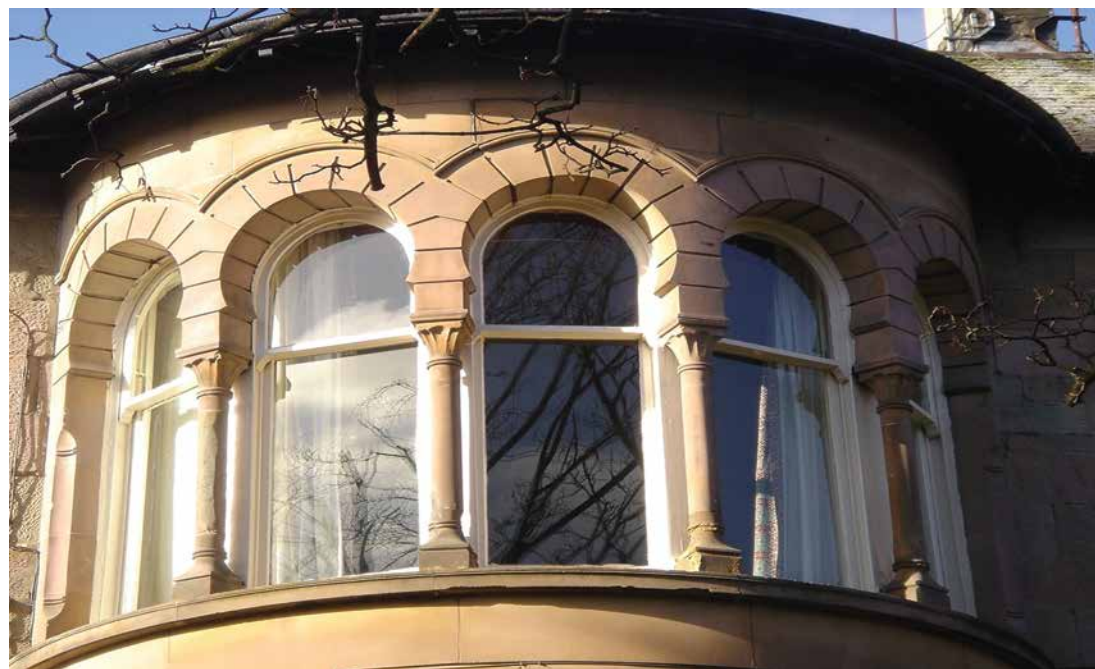
Top left and right: Historic windows before and after repair (courtesy of Glasgow City Heritage Trust) Bottom: West Pollokshields
