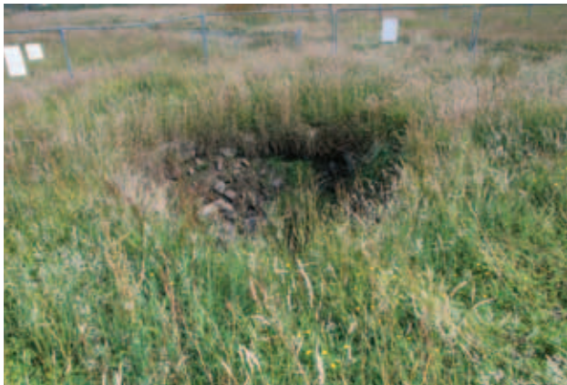
Mining collapse, Castlecary
